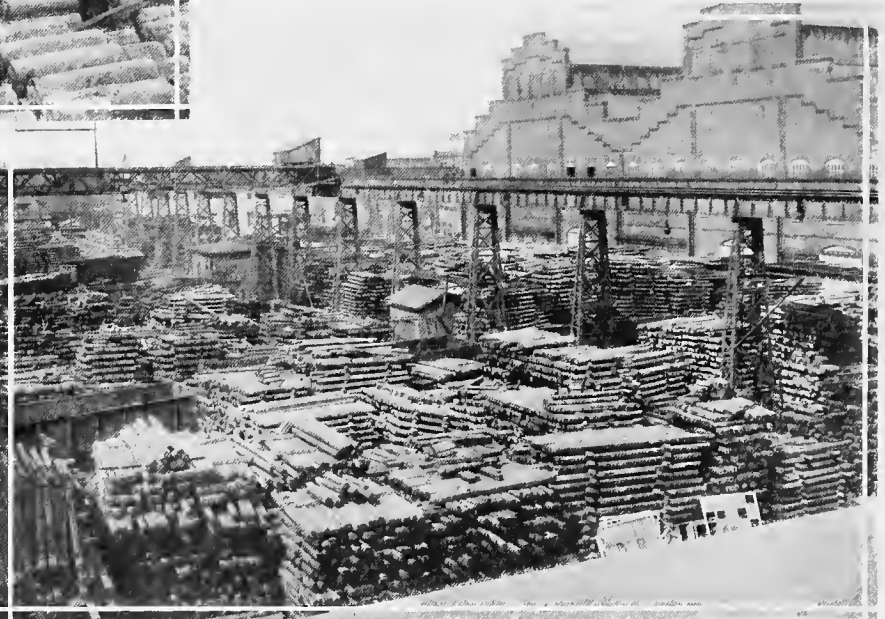
Storage of Steel Billets in Steel Yard for 155 mm. Shell Forgings
